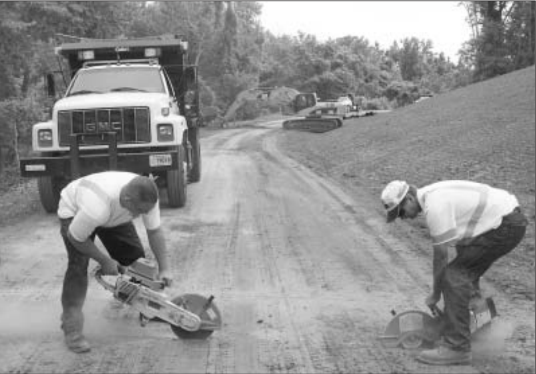
PHOTO BY KEITH TODD Kentucky Transportation Cabinet personnel have been making drainage and safety improvements to Ky. 387/Dam 50 Road in Crittenden County. Several cross drains were added near the entrance to the Dam 50 Riverview Recreation Area over the last week. Above, David West (left) and Darrell Bebout cut out a section of pavement to install a cross drain.
