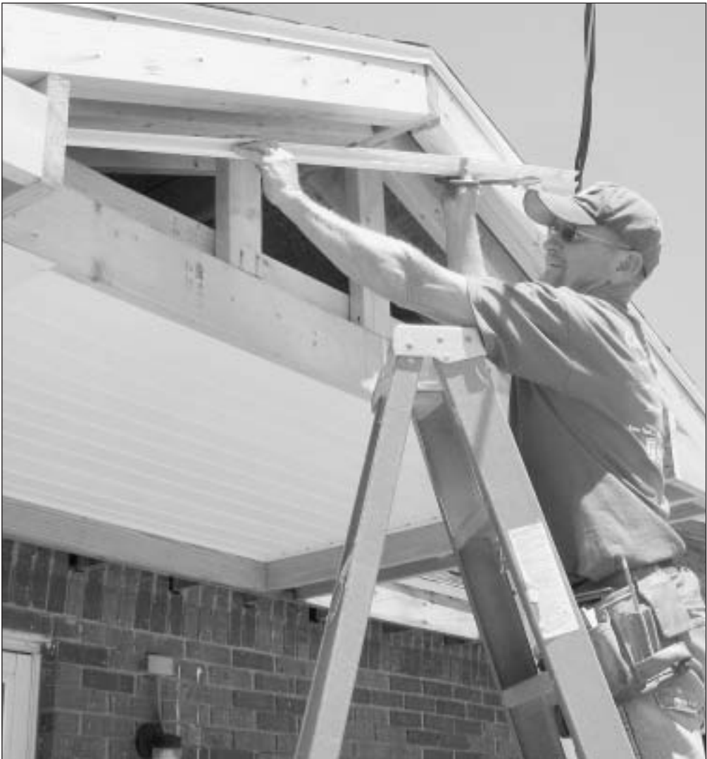
PHOTO BY DARYL K. TABOR David Perryman, a maintenance technician with Crittenden County’s school district, replaces molding Friday along the eve of an overhang at the district’s central office on West Elm Street. The roof of the building is being replaced after last winter’s ice storm and subsequent wind storm compromised its ability to keep out the weather. Because the school district is using its own labor coupled with the insurance settlement, there is no out-of-pocket expense to replace the roof. A larger roofing project just down the hill from the central office is also costing the district nothing from its budget. Workers are currently in the midst of replacing the roof on the high school, music department and old gymnasium, using more that $1 million in state-allocated monies designated solely for capital improvements.
